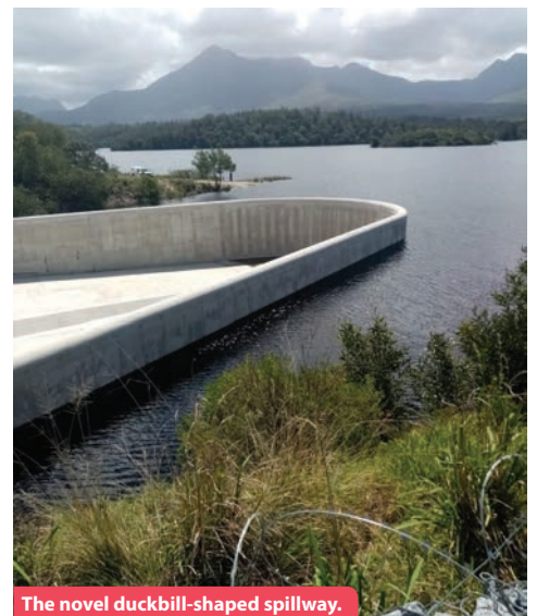
The novel duckbill-shaped spillway.
